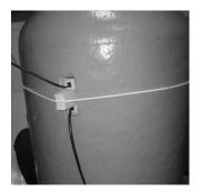
For a daisy chain installation of pipe/ tank sensors, it is important that you do not disturb the slider button positions, otherwise none of any SES 002 sensors will communicate.
